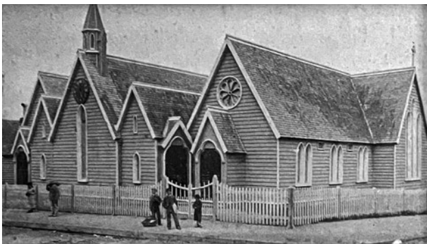
The first St Peter's Church. This picture shows the building as it appeared after four enlargements to the church of 1848. This framed photo was given to the church by the family of a Miss Keap-Read who died in 1942 at the age of 89. According to the inscription she had attended the church from 1865 and was a Sunday school teacher from 1869. The frame of the photo is made from the foundations of the original building.
